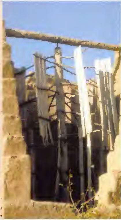
Left to right: 14 th century manuscript by al-Dimashqi showing the cross section of a windmill whose vertical vanes rotate around a vertical shaft; an old windmill in Herat, Afghanistan.
